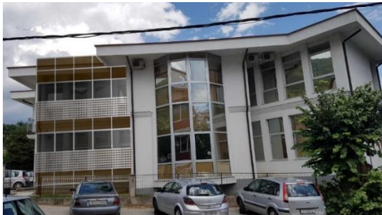
Figure 6: Appearance of the North Facade of the Regional and Local Administration Building located in Zhelino: a partially coated double facade with integrated photovoltaic panels of system A
