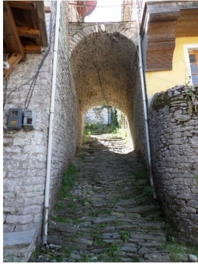
Figure 17: Tunnel connecting the building with the other part
