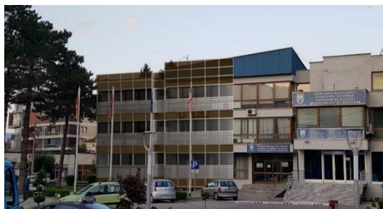
Figure 4: Appearance of the west facade of Regional and Local Administration Building located in Gostivar: provided (partly coated) double facade panels with integrated photovoltaic system A
