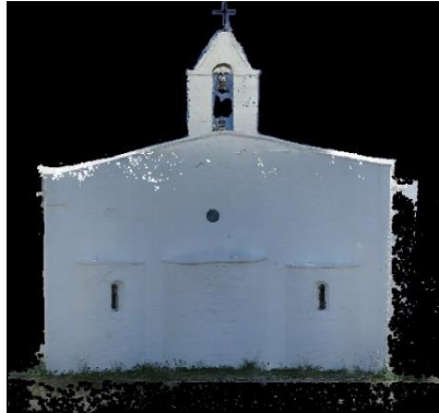
Figure 3: photopiano processing of the church of San Michele in Frangesto, Fasano | rearward prospectus
