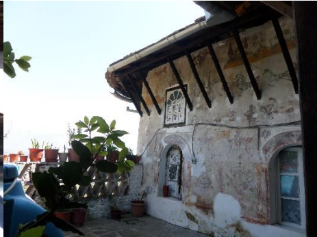
Figure 30: Roof construction element in Zekate House
