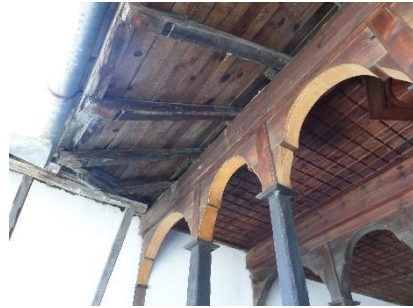
Figure 25: Roof construction element in Zekate House
