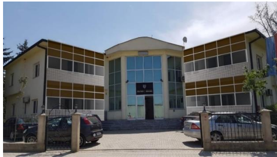
Figure 8: Appearance of the southern façade of the Regional and Local Administration Building located in Tearce: provided (partially coated) double facade with integrated photovoltaic panels of system B
