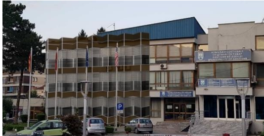
Figure 5: Appearance of the southern façade of the Regional and Local Administration Building located in Tearce: provided (partially coated) double facade with integrated photovoltaic panels of system A
