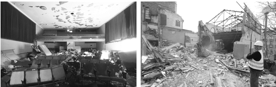
Figure 3: 2014, demolition of the old Parochial Hall.
