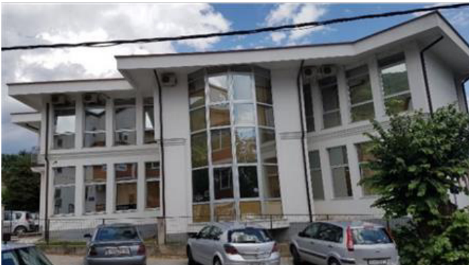
Figure 2: Regional and Local Administration Building located in Tearce, south façade (photographed: 08.08.2017.)
