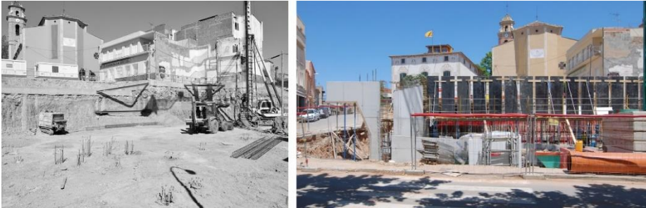
Figure 4: Retaining wall constructed by piles and early stages of the new Hall.
