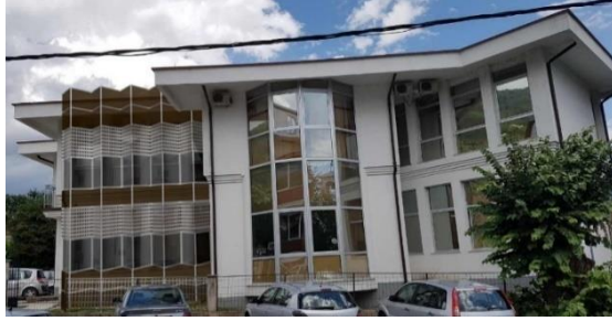
Figure 7: Appearance of the west façade of Regional and Local Administration Building located in Gostivar: provided (partly coated) double facade panels with integrated photovoltaic system B
