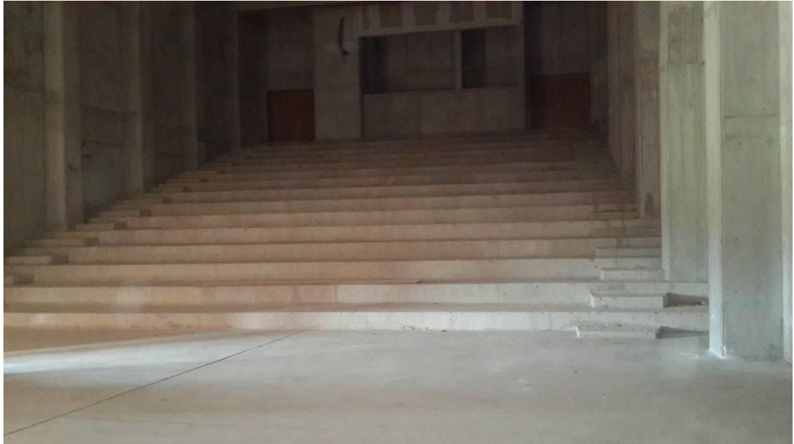
Figure 20 View from Conference Hall 2, under construction
